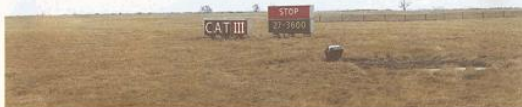
Figure A-4. A Category III taxi-holding position and a stop sign installed side by side
